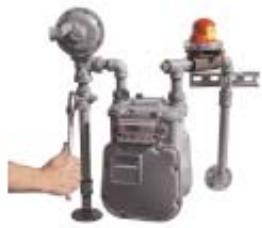
14. Turn gas on at meter inlet valve, **do not** use pipe wrench. Note: Open gas valve slowly to prevent damage to regulator.
