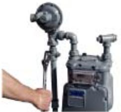
2. Turn gas off at meter inlet valve, **do not** use a pipe wrench.
