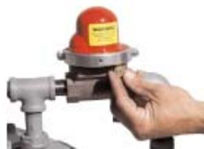
13. While gas is **still off**, open seismic valve. **Do not** open against gas pressure.
