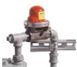
12. Finish meter plumbing system with PSP seismic valve.
